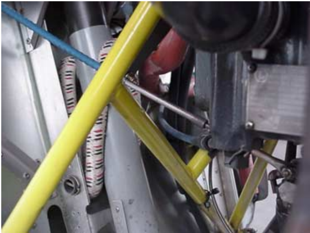
Cable routing under oil pan
