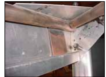
3 RIVETS A5 In front steel tab welded on the cabin frame
