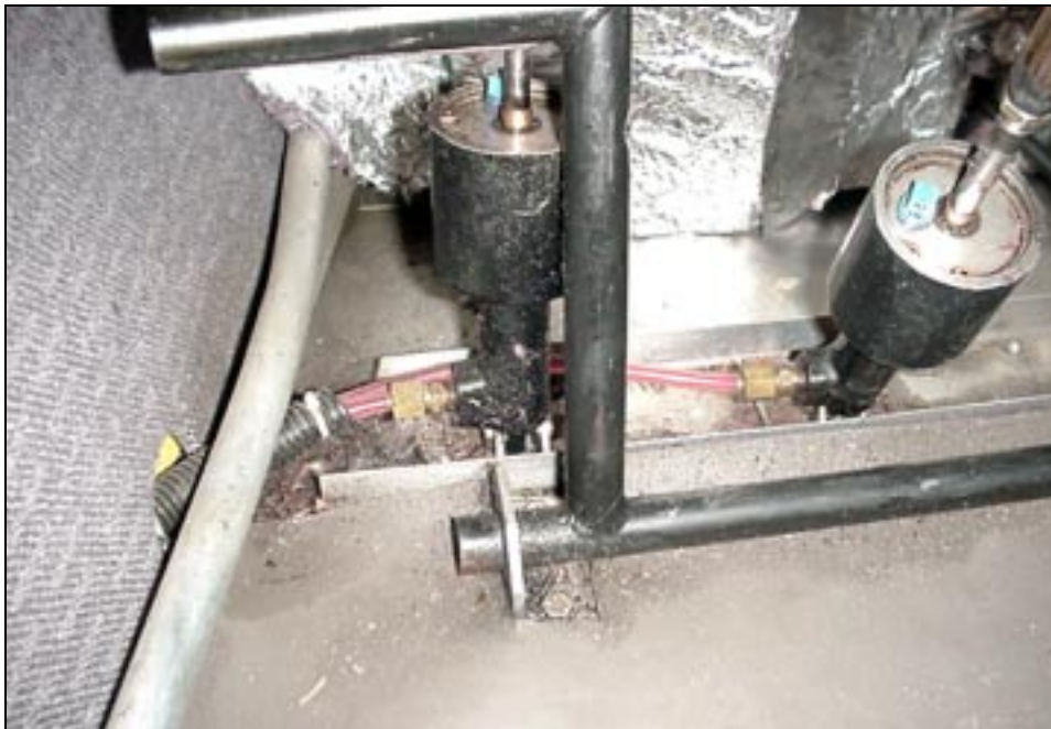
Fittings out outboard side of master cylinders.
